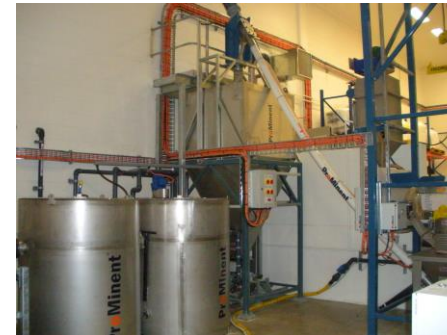
Bulk Bag Fluoride Package using Flexicon bag unloader
