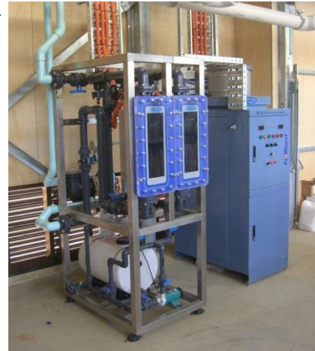
Electrochlorinator Chlorine from salt
